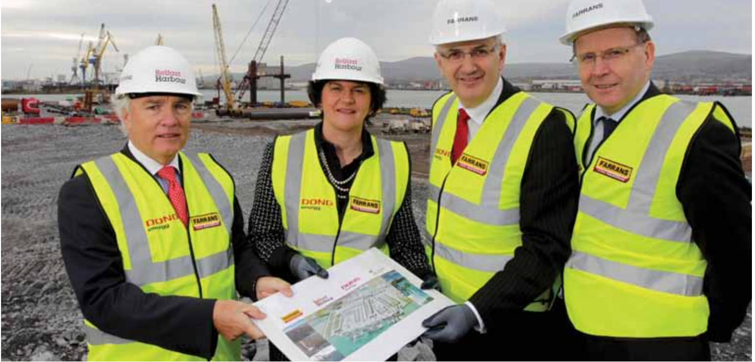
Len O'Hagan, Chairman, Belfast Harbour, DETI Minister Arlene Foster, DRD Minister Danny Kennedy and Eamonn Sweeney, Farrans MD, on a recent visit to the site where the assembly of offshore wind turbines will be undertaken.
