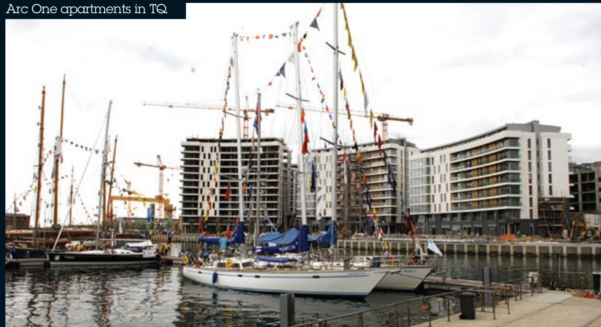
Arc One apartments in TQ
