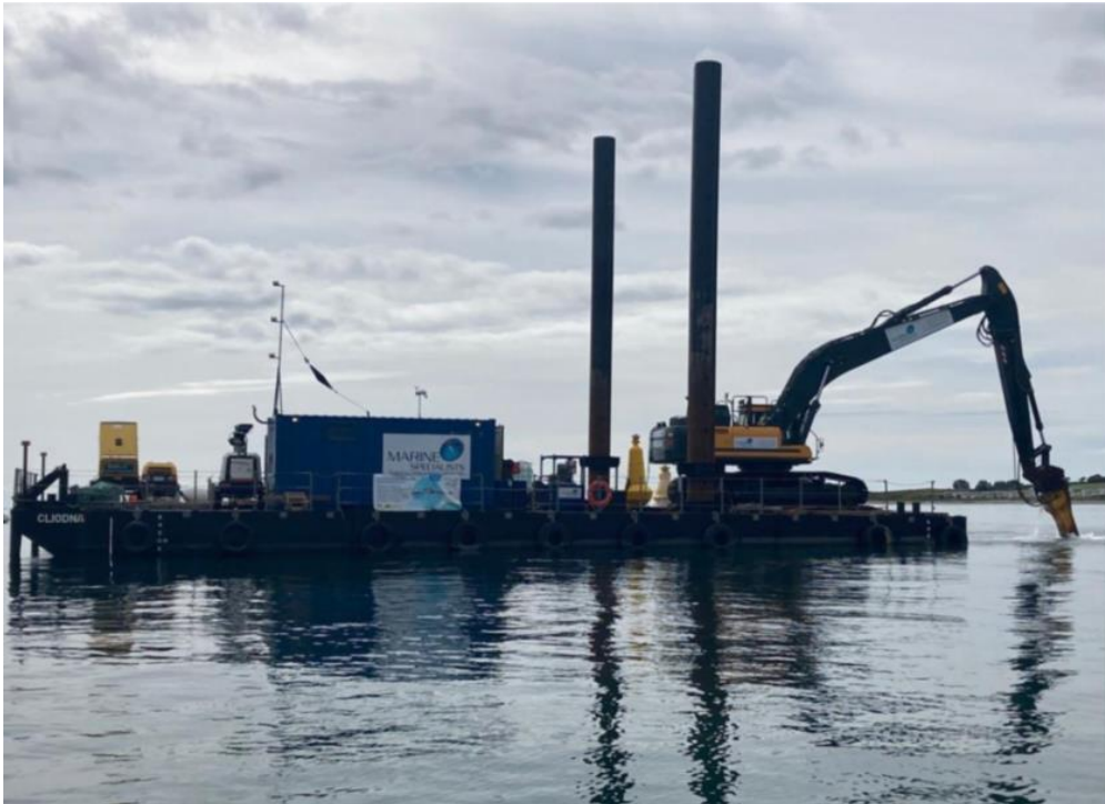
Figure 3: Marine Specialists pontoon barge – Clidna
