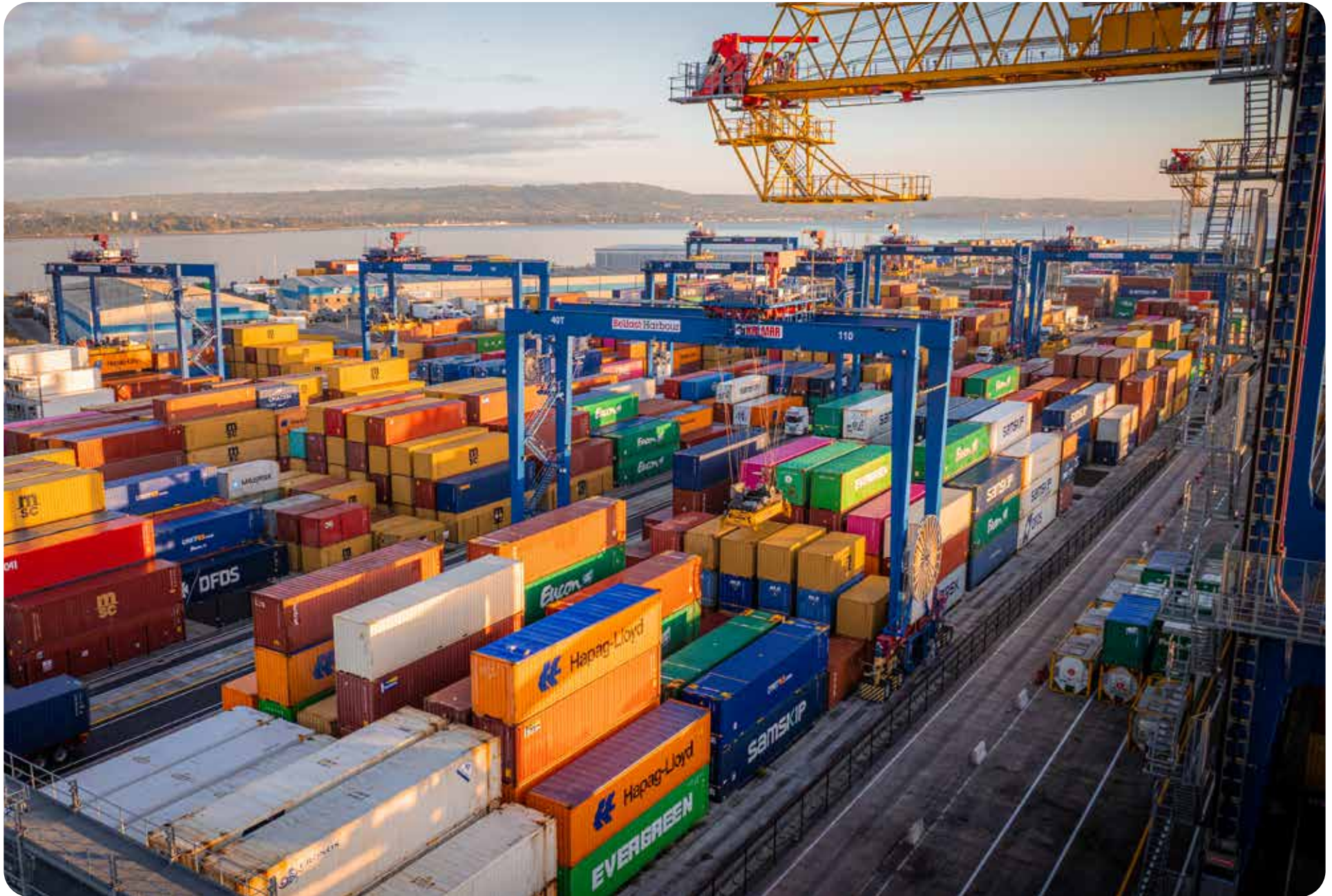
Victoria Terminal 3 (VT3) Container Port
