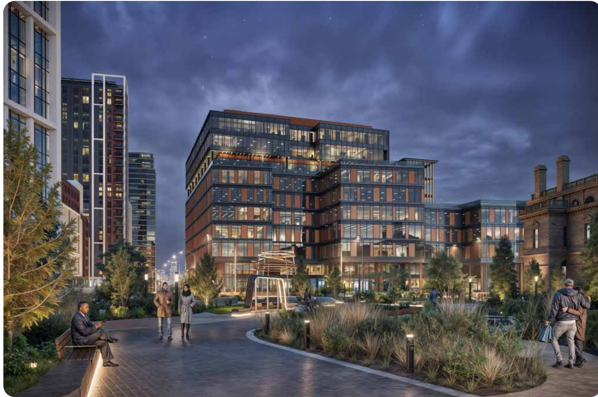
Architect's visualisation of City Quays 5, viewed from City Quays Gardens.
