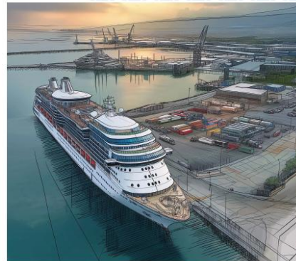
Artist's impression of a dual-purpose deepwater quay in use as a cruise terminal
